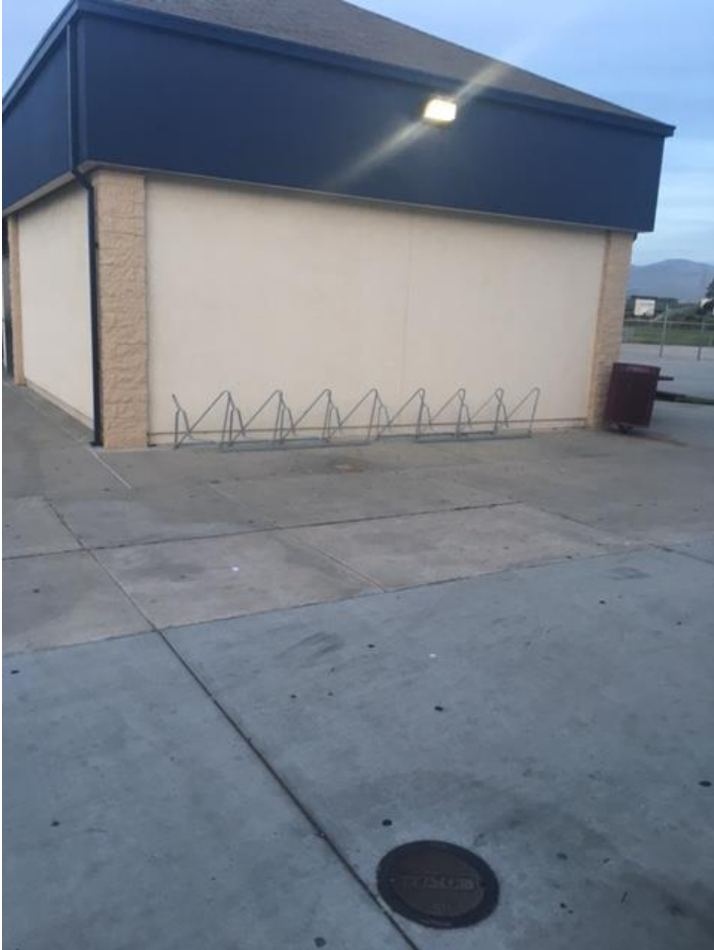
Figure 6 Everett Alvarez High School Bike Racks
