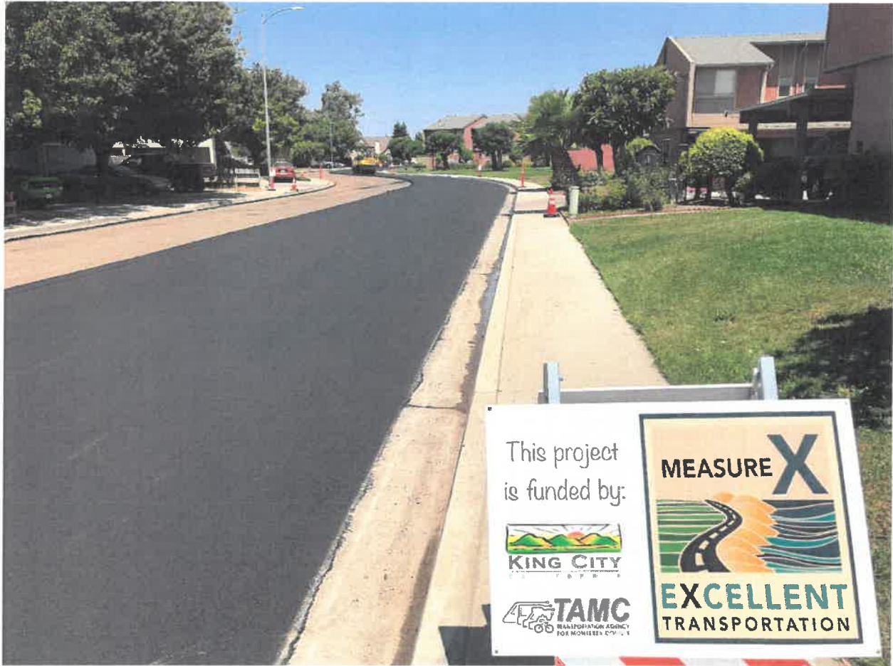
Figure 2 Repaving Bishop Street
