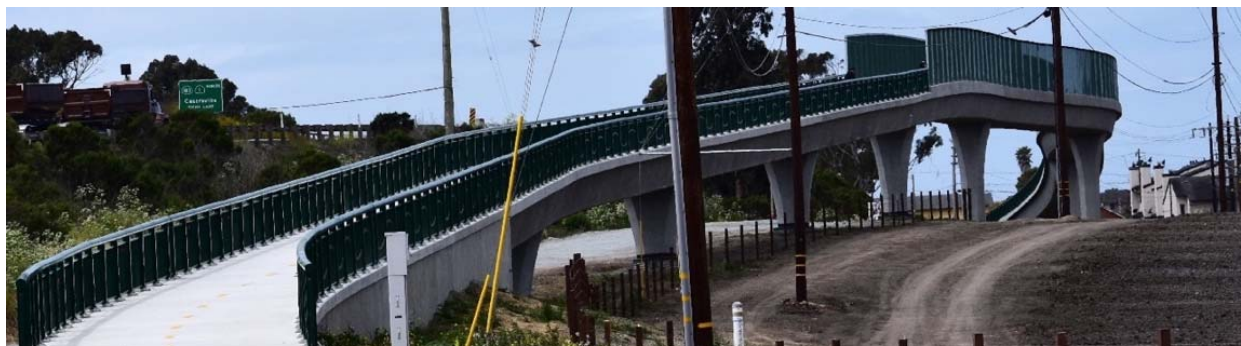
Castroville Bike/Ped Bridge
