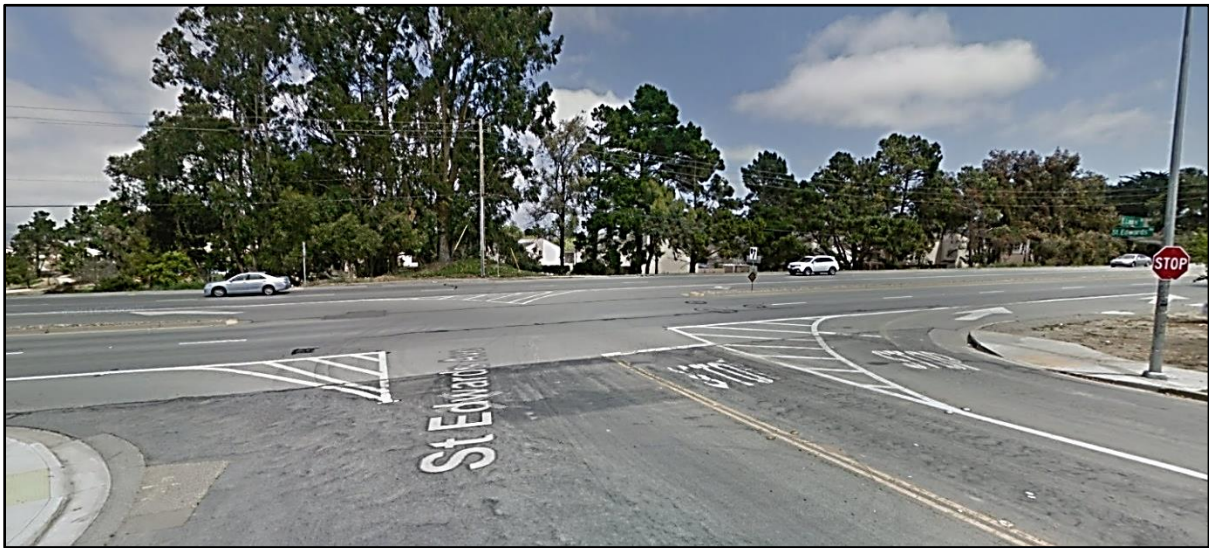
St. Edwards Dr. at E. Laurel Dr. before traffic signal installation.
