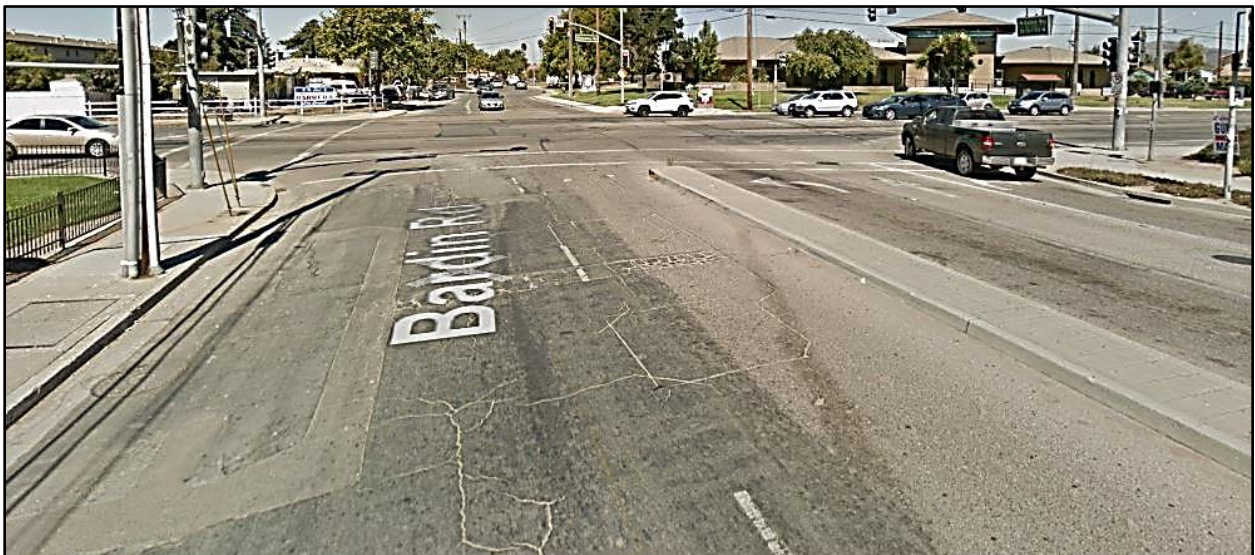
Before photo of Bardin Rd at Williams Rd
