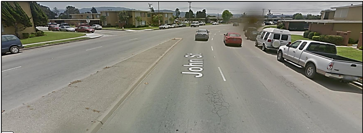
Before photo of John St between Williams Rd and John Cir
