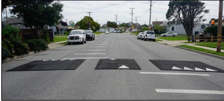
West Curtis Street- After with Traffic Calming (speed cushions)
