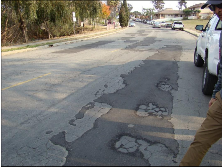
Circle Drive – before slurry seal
