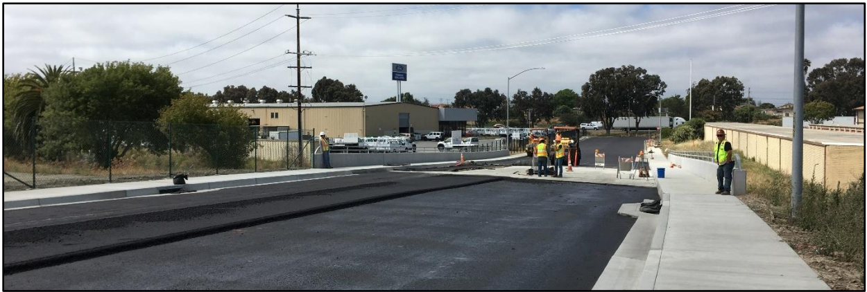
Elvee Drive near bridge construction
