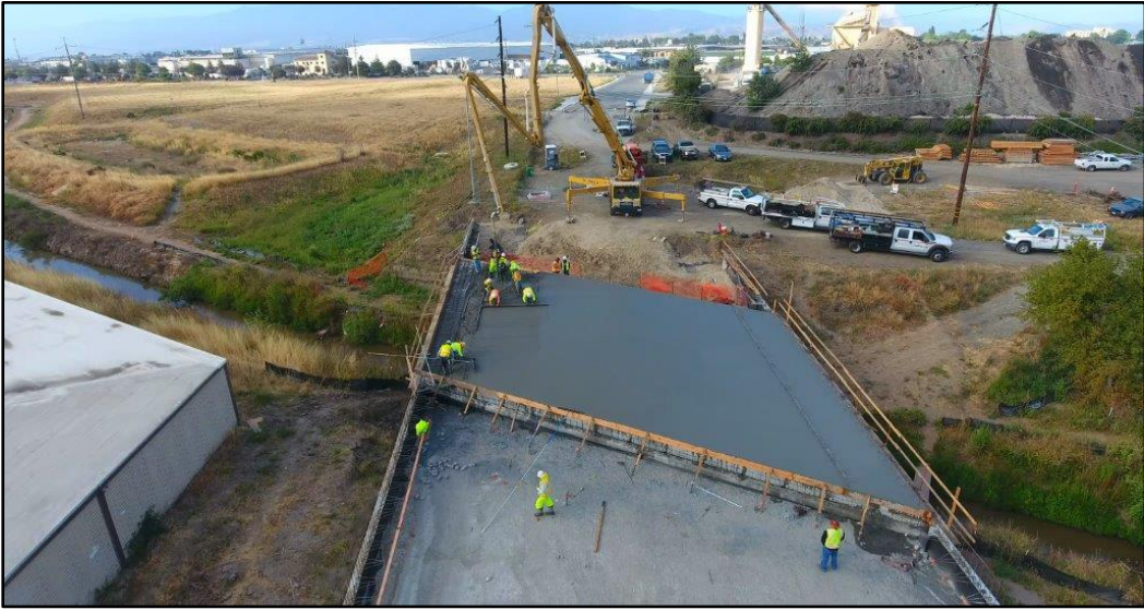
Construction of bridge at Elvee Drive
