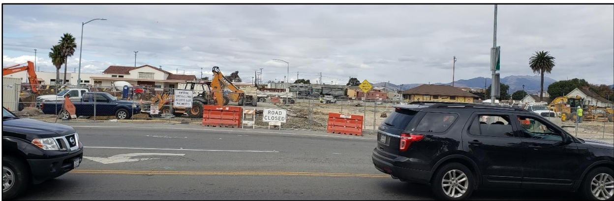
ITC Construction, view from Lincoln Avenue
