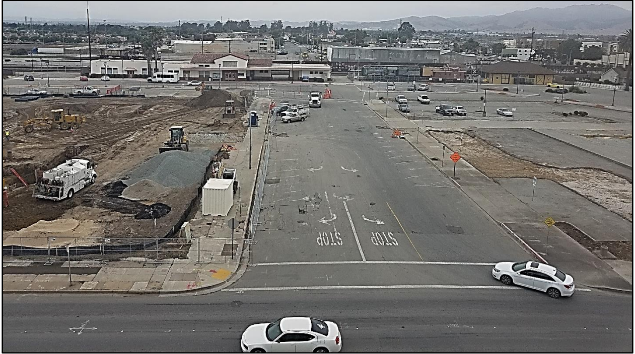
Station Place at Lincoln Avenue
