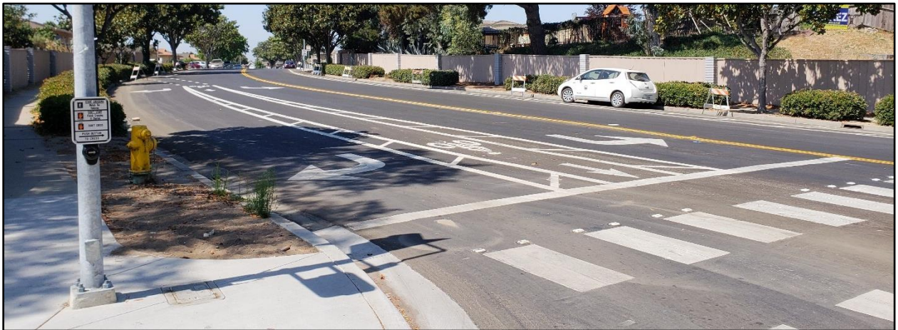
St. Edwards Dr. at E. Laurel Dr. after traffic signal installation.
