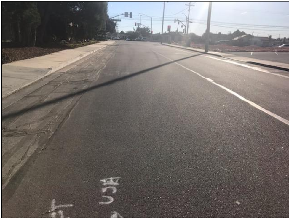
Circle Drive – after slurry seal
