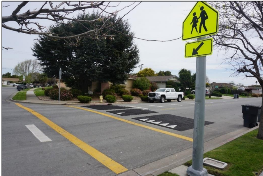
Ambrose Drive- After with Traffic Calming (speed cushions)
