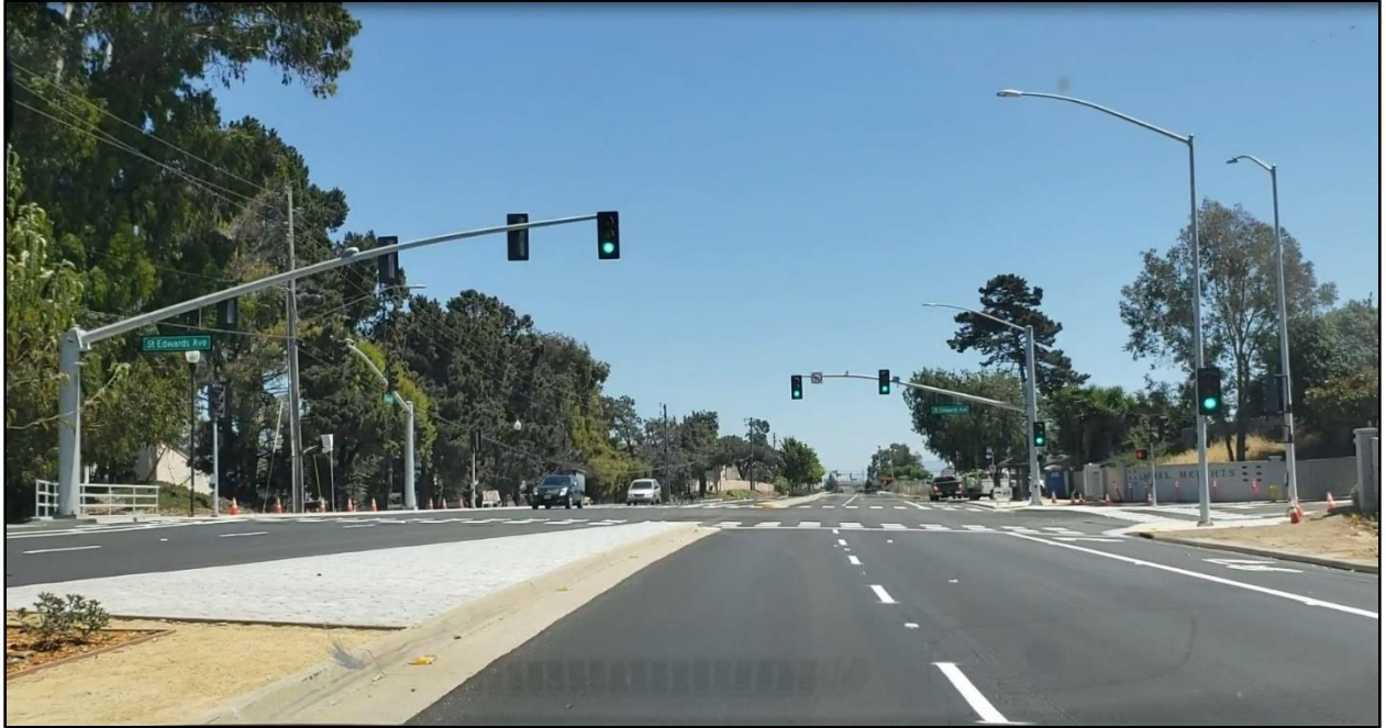
E. Laurel Dr. at St. Edwards Dr. after traffic signal installation.
