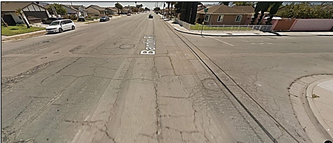
Before photo of Bardin Rd at Afton Rd
