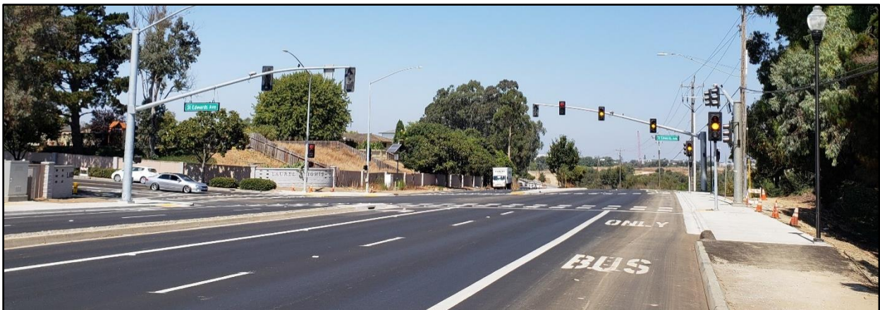
E. Laurel Dr. at St. Edwards Dr. after traffic signal installation
