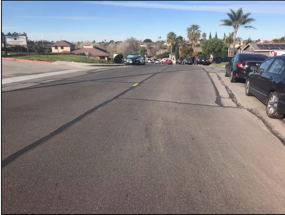
Circle Drive – after crack seal
