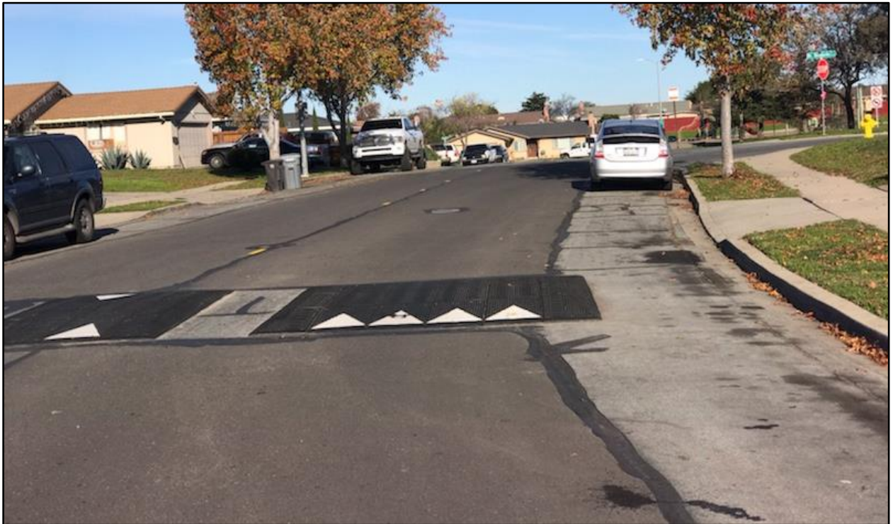
Circle Drive – after crack seal
