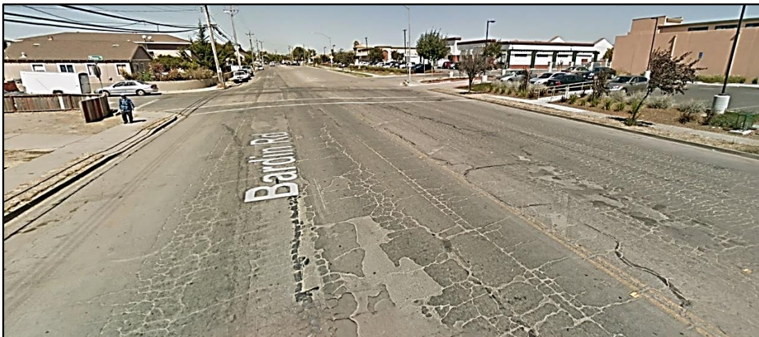
Before photo of Bardin Rd at Toro Ave
