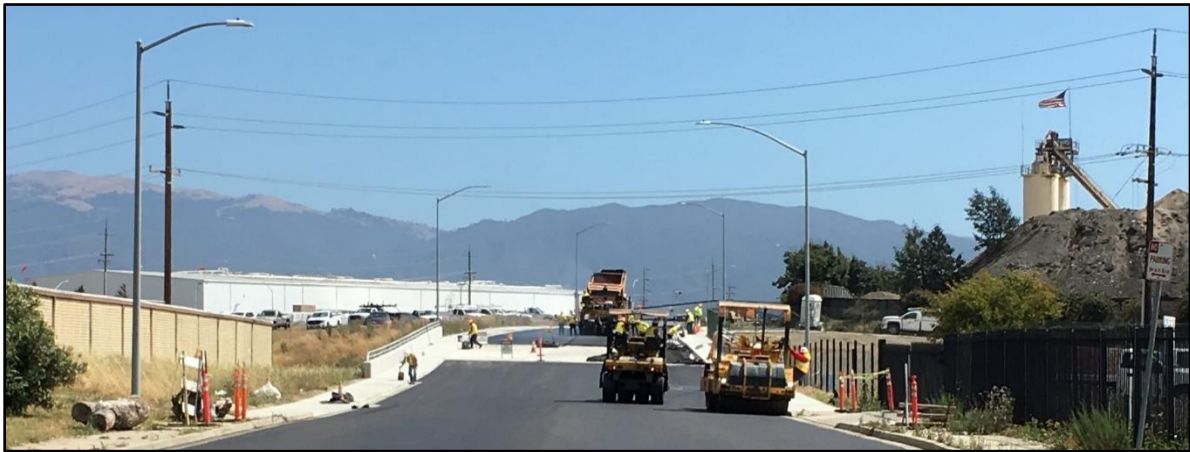
Elvee Drive near bridge construction
