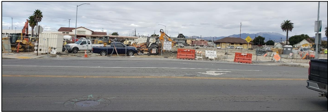
ITC Construction, view from Lincoln Avenue
