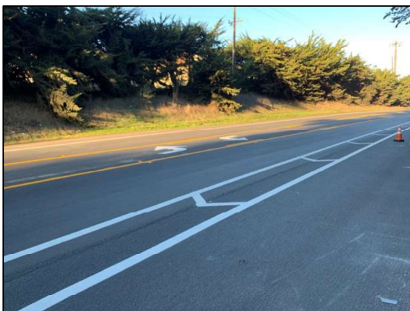
Two Way Left Turn Lane
