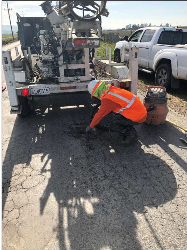
Coring on Old Stage Road
