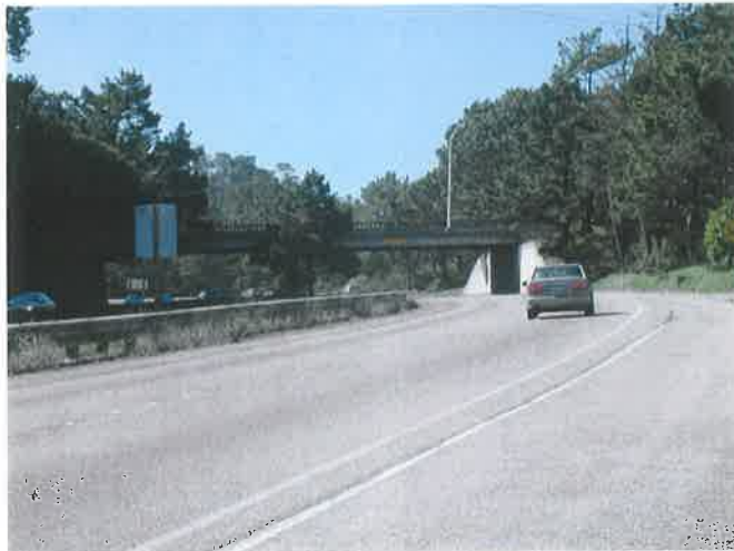
SR 1 Southbound at SR 68 Overcrossing, View to the South
