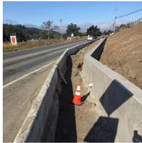
Barrier to retain future erosion
