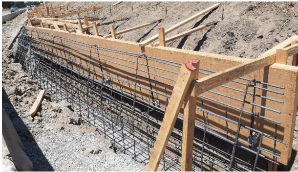
Rebar & form operation
