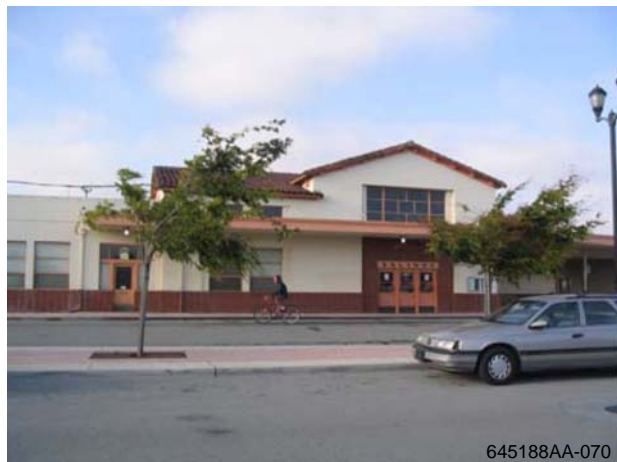
Figure 5-5 Salinas Amtrak Station
