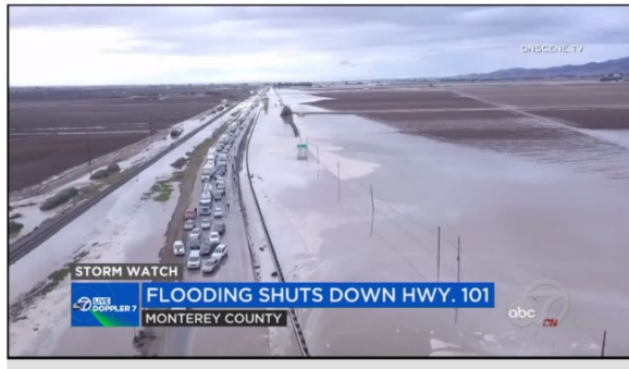
FIGURE 18: IN EARLY DECEMBER 2019, FLOODING SHUT DOWN US 101 AND DRIVERS WERE STUCK FOR HOURS. SOURCE: ABC 7 NEWS (DECEMBER 5, 2019).
