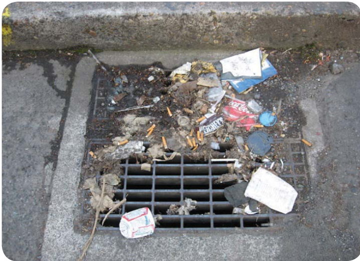
Figure 3: An example of the type of trash that can clog inlets and pollute water bodies (Nevue Ngan Associates)
