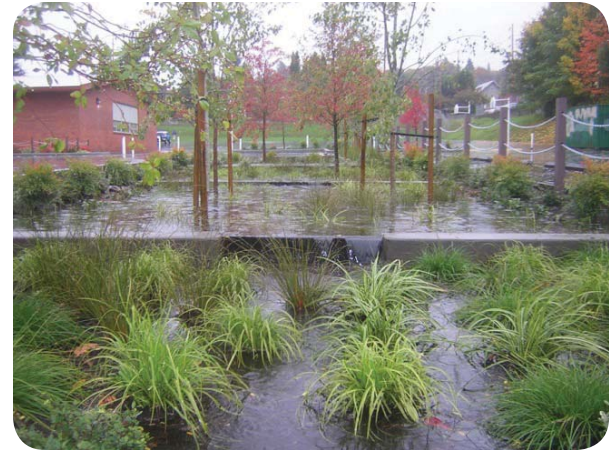
Figure 7: Stormwater facilities slow the flow of stormwater runoff through the interaction of the water with plants and soil (Nevue Ngan Associates)
