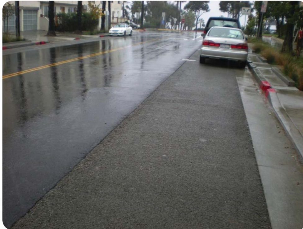
Figure 15: Permeable concrete after a rain event (Neil Shapiro)
