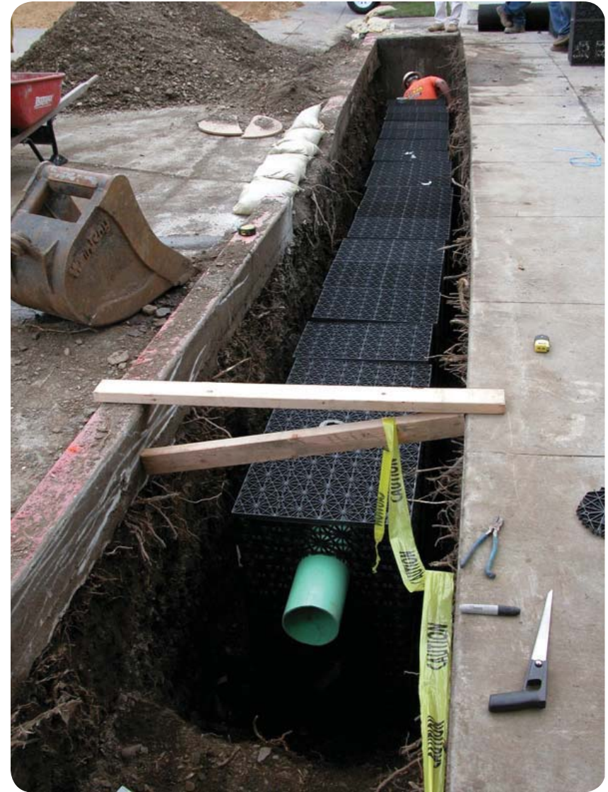
Figure 19: Infiltration trench with perforated pipe during installation (Neil Shapiro)
