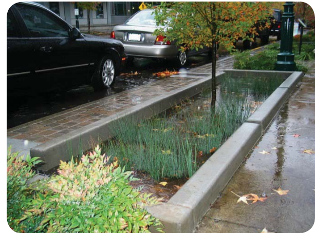
Figure 8: Stormwater facilities collect and absorb stormwater to reduce the overall volume of runoff (Kevin Robert Perry – City of Portland)
