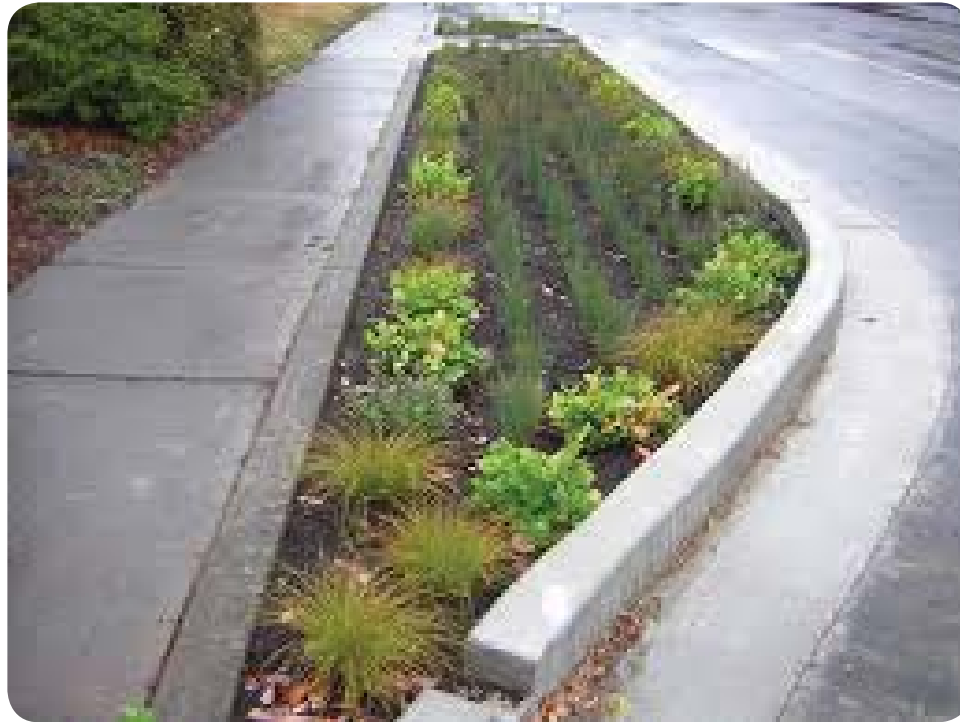
Figure 14: Stormwater curb extension (Kevin Robert Perry – City of Portland)
