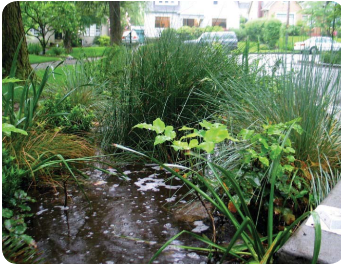
Figure 5: Landscape-based stormwater facilities, such as this stormwater curb extension, can capture urban debris before it gets into creeks and other waterways (Kevin Robert Perry – City of Portland)
