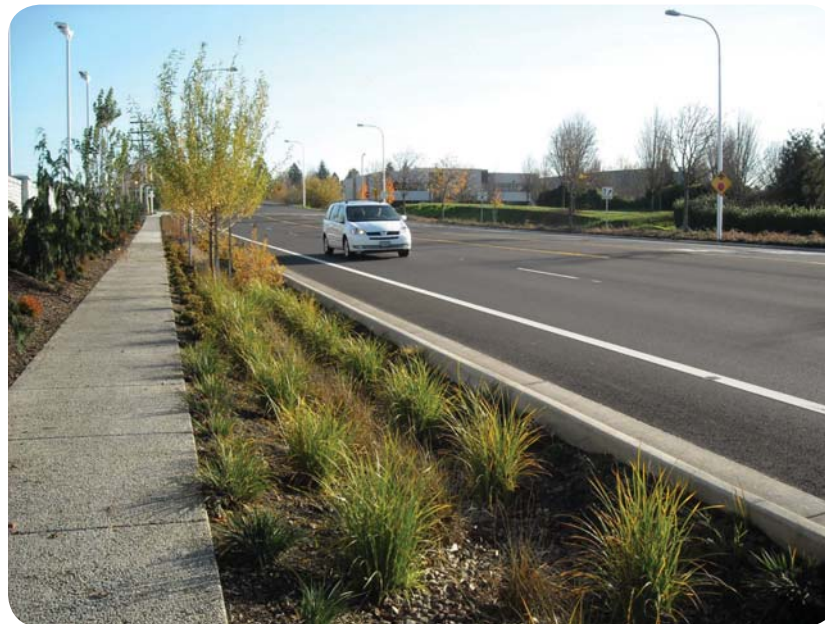
Figure 1: The green street utilizes a vegetated swale to accept stormwater from the street. It also uses sidewalks made from pervious concrete. (Nevue Ngan Associates)
