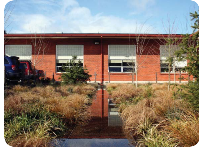
Figure 6: Stormwater facilities filter sediments and other pollutants in runoff; which results in improved water quality (Kevin Roberts Perry – City of Portland)
