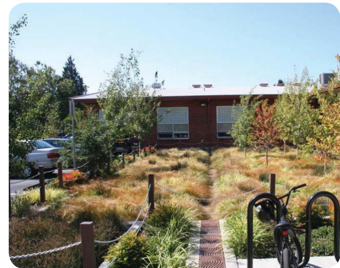
Figure 13: This rectangular rain garden area receives runoff from both a parking lot and the building’s rooftop (Nevue Ngan Associates)
