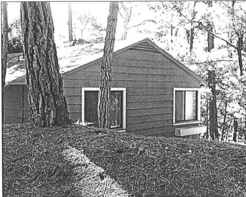
View E, 5/21/03, filename: PIC00008.jpg, Accession #02-1006-dig-2
