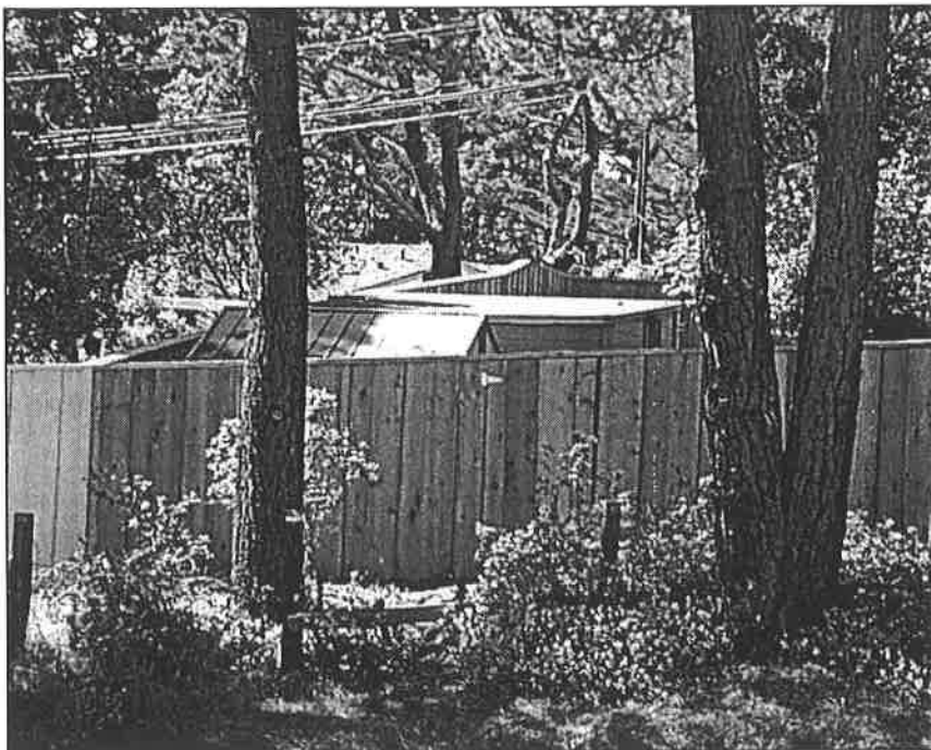
Outbuilding; View SW, 10/10/02, filename: PIC00026.jpg, Accession #02-1006-dig-1
